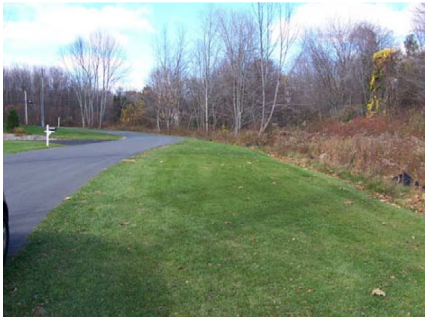
Figure 3-2: Example of a Vegetative Filter Strip (Figure 4.6.1 from Low Impact Development SWM Planning and Design Guide, 2010 )
