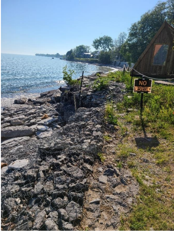
Figure C3 – Centre of gabion wall facing west.
