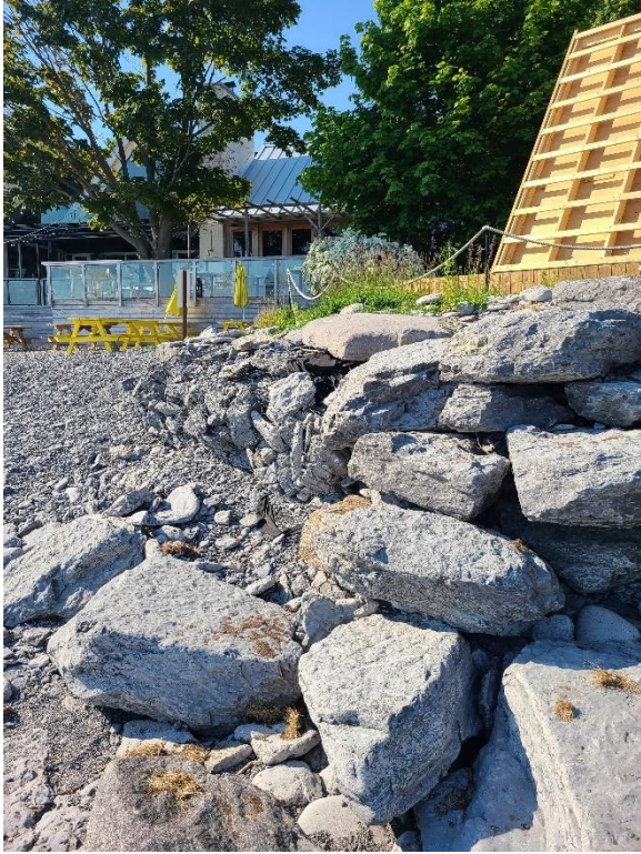
Figure C1 – West end of gabion wall facing Drake Devonshire rear beach.
