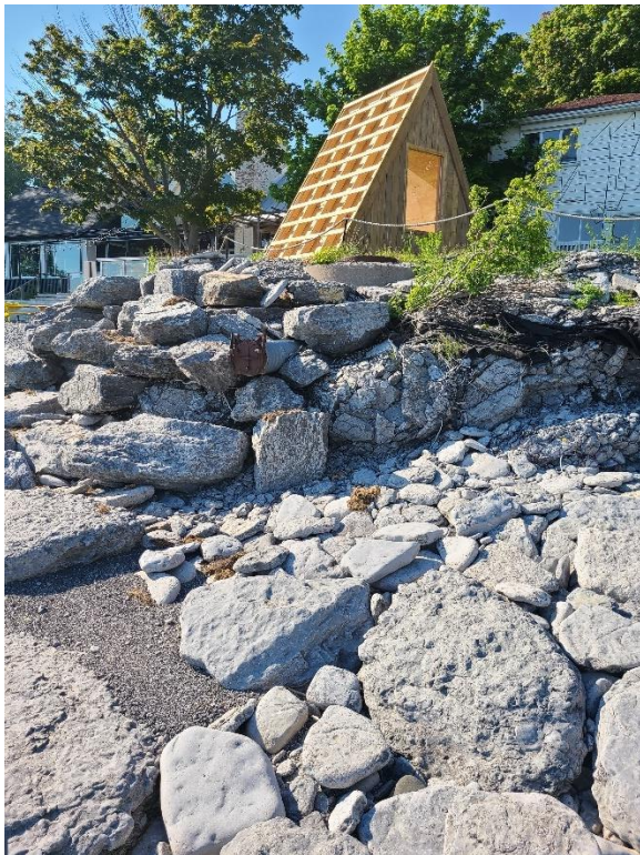
Figure C2 – West end of gabion wall facing northwest, with manhole and culvert.
