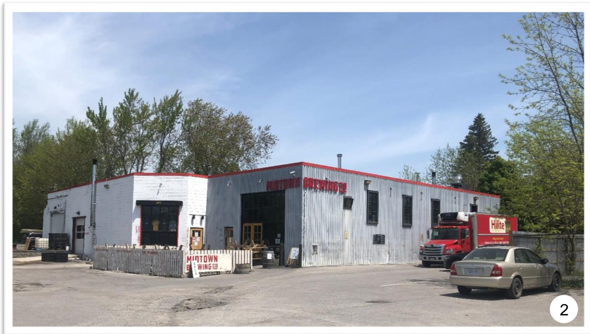
Looking north-east at Midtown Brewing Company site (former Midtown Meats; 266 Main Street)
