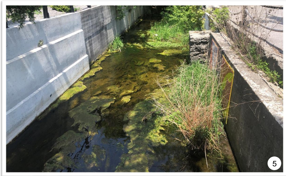
View looking north of Lane Creek bordered by concrete retaining walls
