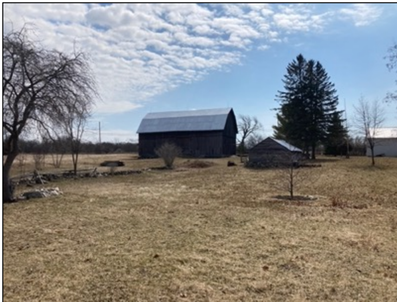
Image 6: Shows existing structures and conditions for test pit survey.
