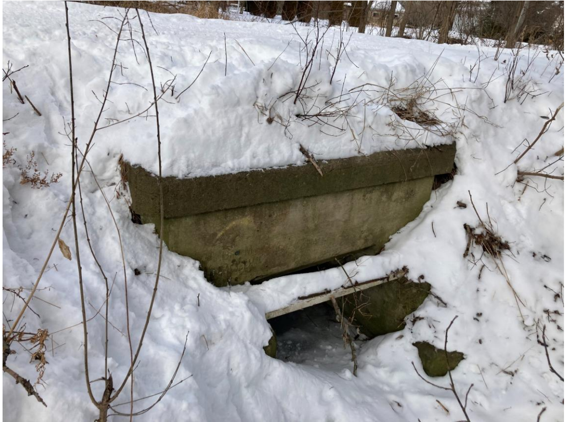
Photo 9: Box culvert in northeastern portion of study area (January 30, 2022)
