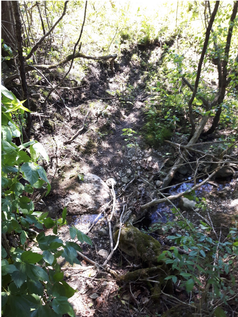
Photo 15: view of the west flowing drainage ditch observed along the north property limit of the Phase One Property, viewing west
