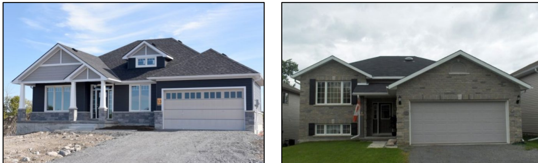
Figure 27 Sample Building Exterior - Antonia Heights, Quinte West (Hilden Homes)
