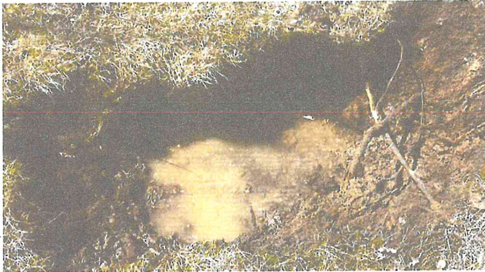
Photo 4 – Example of seepage near ground level due to underlying bedrock.
