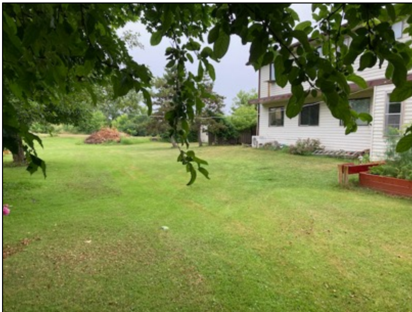
Image 4: Shows existing structure and conditions for test pit survey.
