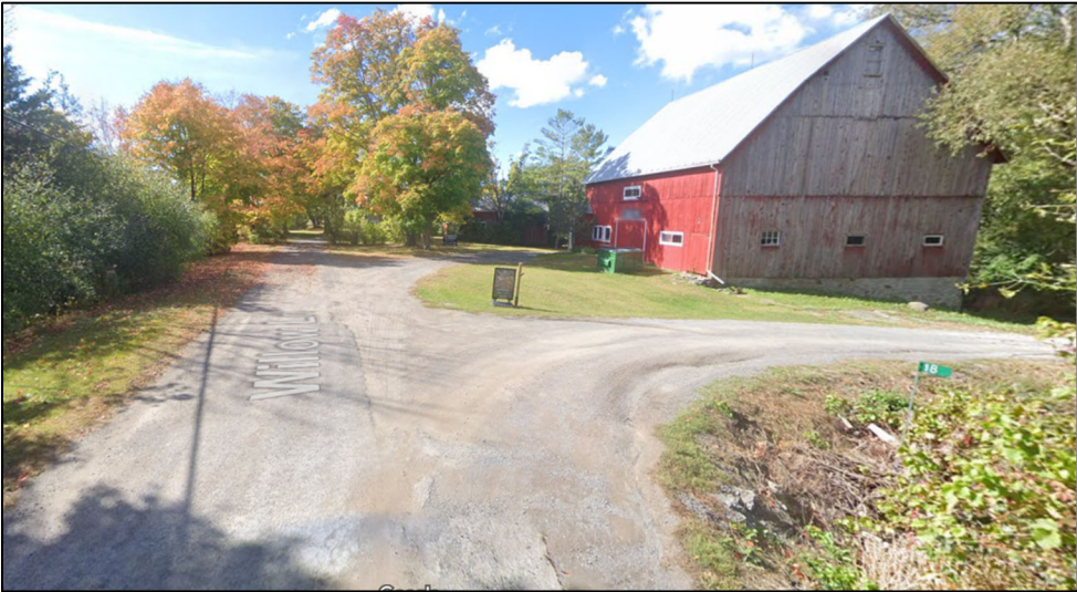
Figure 3: Looking west (Google 2023) from Willow Lane towards: Residential Entrance, in front of the barn. Commercial Property Entrance, behind the barn. Residential Entrance, straight.
