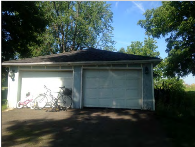
Photo 2 – Site Building B (east elevation).
