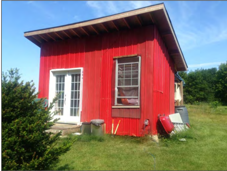
Photo 3 – Site Building C (south and east elevations).
