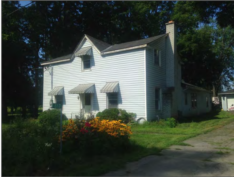
Photo 1 – Site Building A (north and east elevations).
