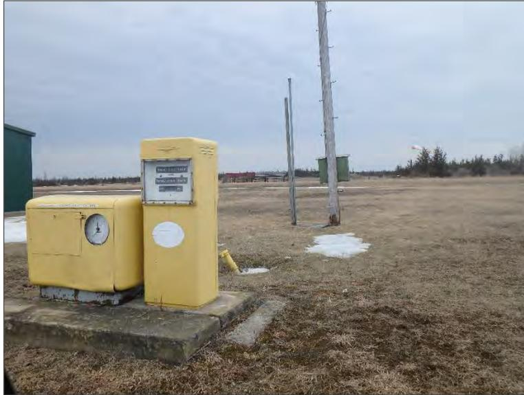
Photo 23 – Gasoline UST and fuel dispenser located west of Site Building 19.
