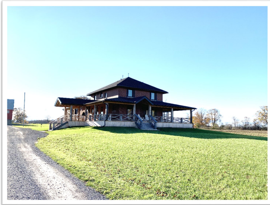
3131 Victoria Road – View of existing two-storey dwelling looking south.
