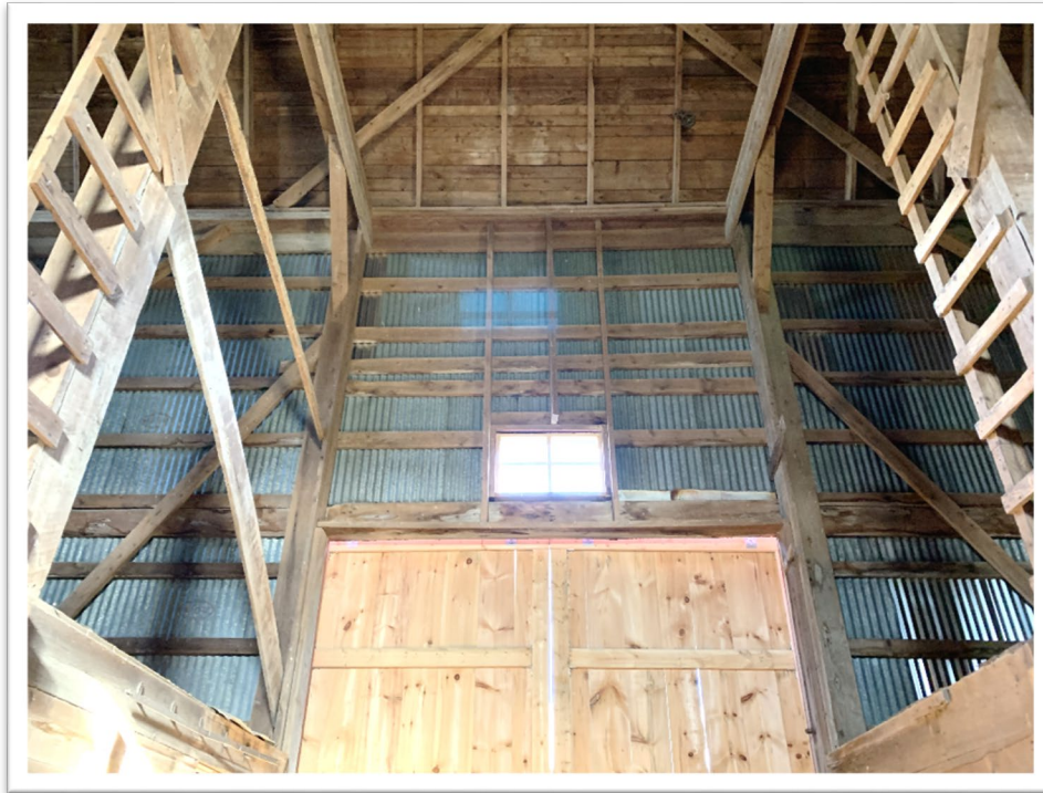
3131 Victoria Road – Interior view of barn loft.
