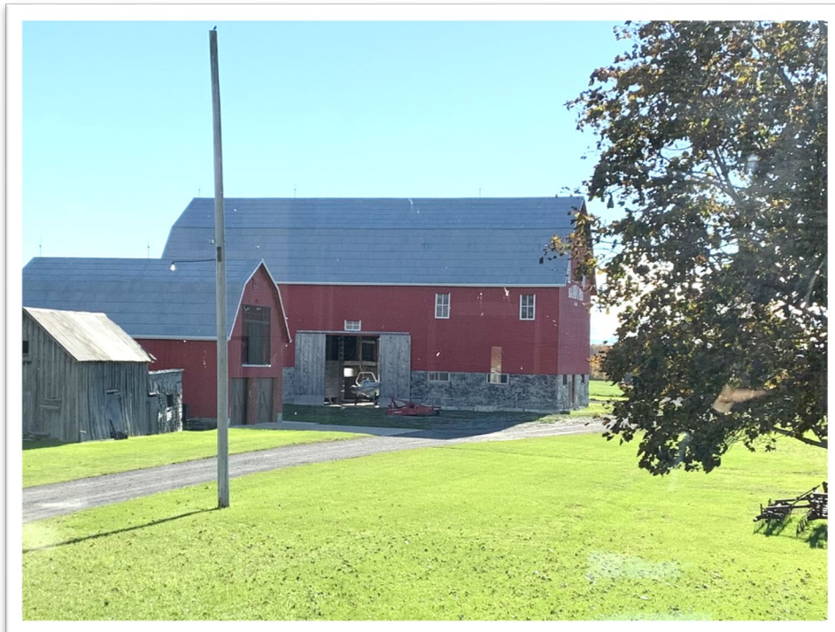
3131 Victoria Road – View of existing two-storey garage and barn looking south.
