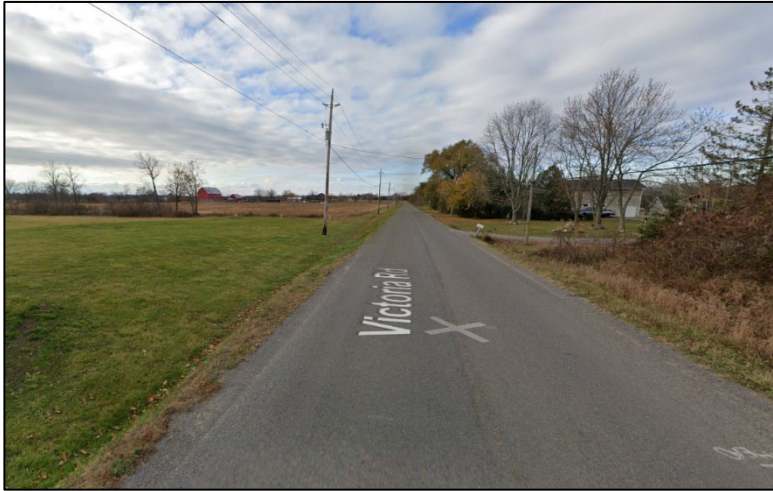
Figure 8.5: Looking South on Victoria Road ~320m from 3131 Victoria Road
