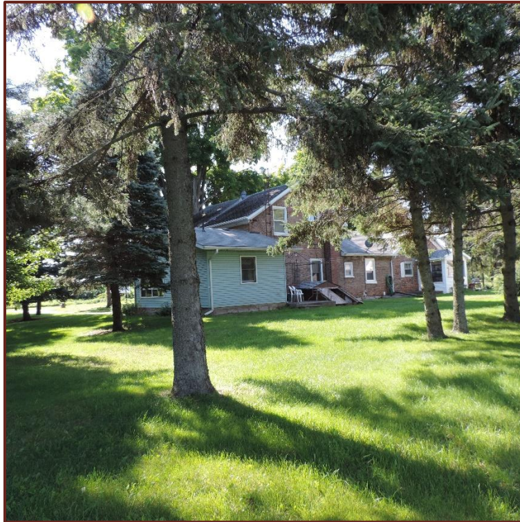
Photo 3. A view of the back of the existing dwelling (August 22 nd , 2023).
