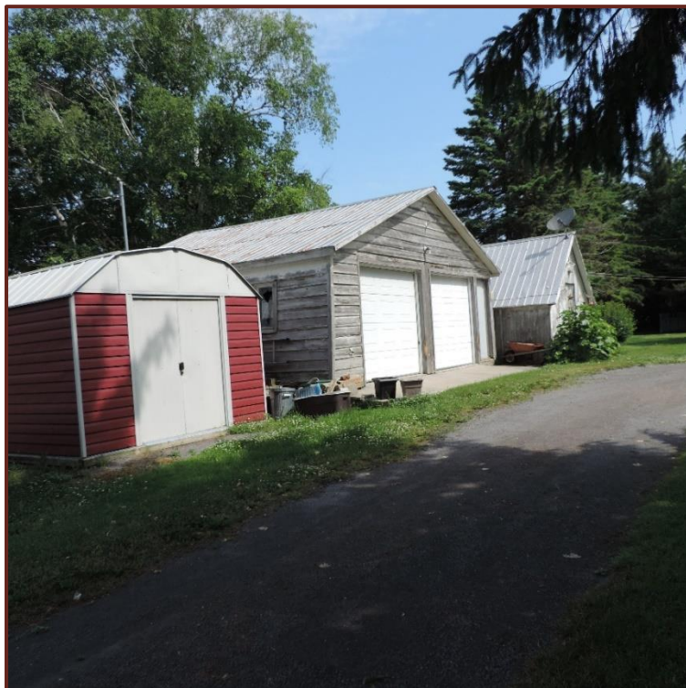
Photo 4. A view of the sheds located around the dwelling (June 15 th , 2023).
