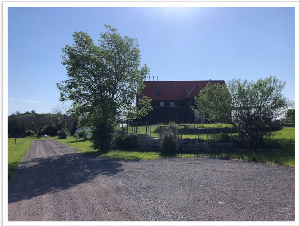
Photo 5 – Existing on-farm diversified use building.
