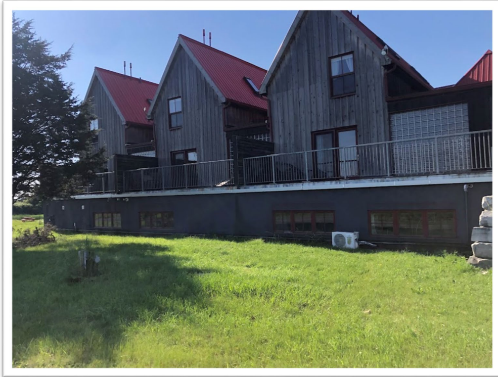
Photo 6 – Front of existing on-farm diversified use building.
