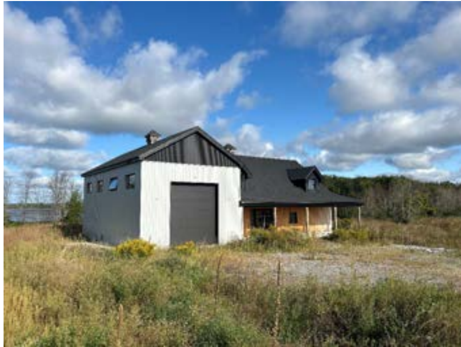
Photo 1 Looking north at building, September 2023.
