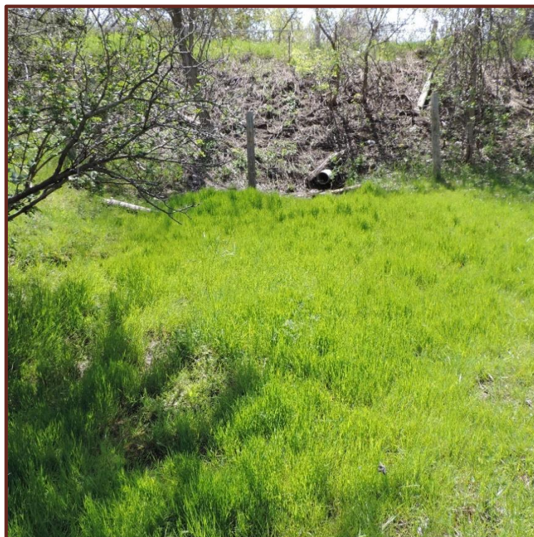
Photo 16. A view of the culvert under County Road 22 and Marsh Creek in the property.
