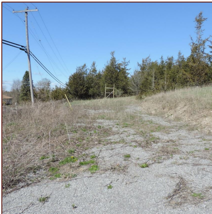
Photo 2. A view of the area adjacent to the driveway where the natural soil and bedrock have been removed.
