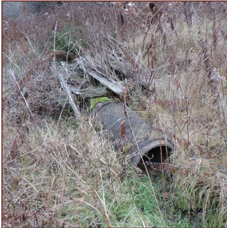
Photo 9. A view of the culverts and old wood bridge found in the creek.
