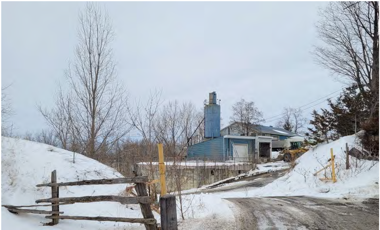
Photo 4: Industrial Concrete Manufacturing facility (Power Concrete products) at 226 Upper Lake Street
