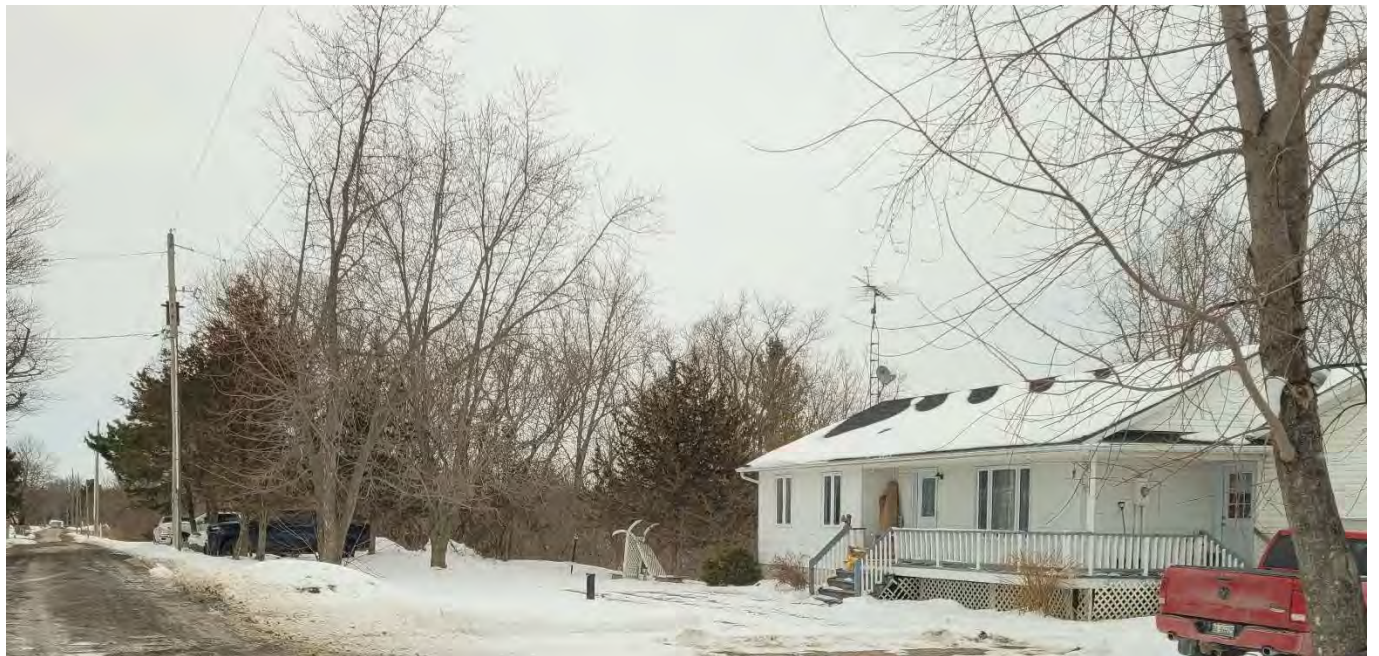
Photo 8: A water supply well located at 229 Upper Lake Street with a hydro pole mounted transformer located in the left portion of the photograph
