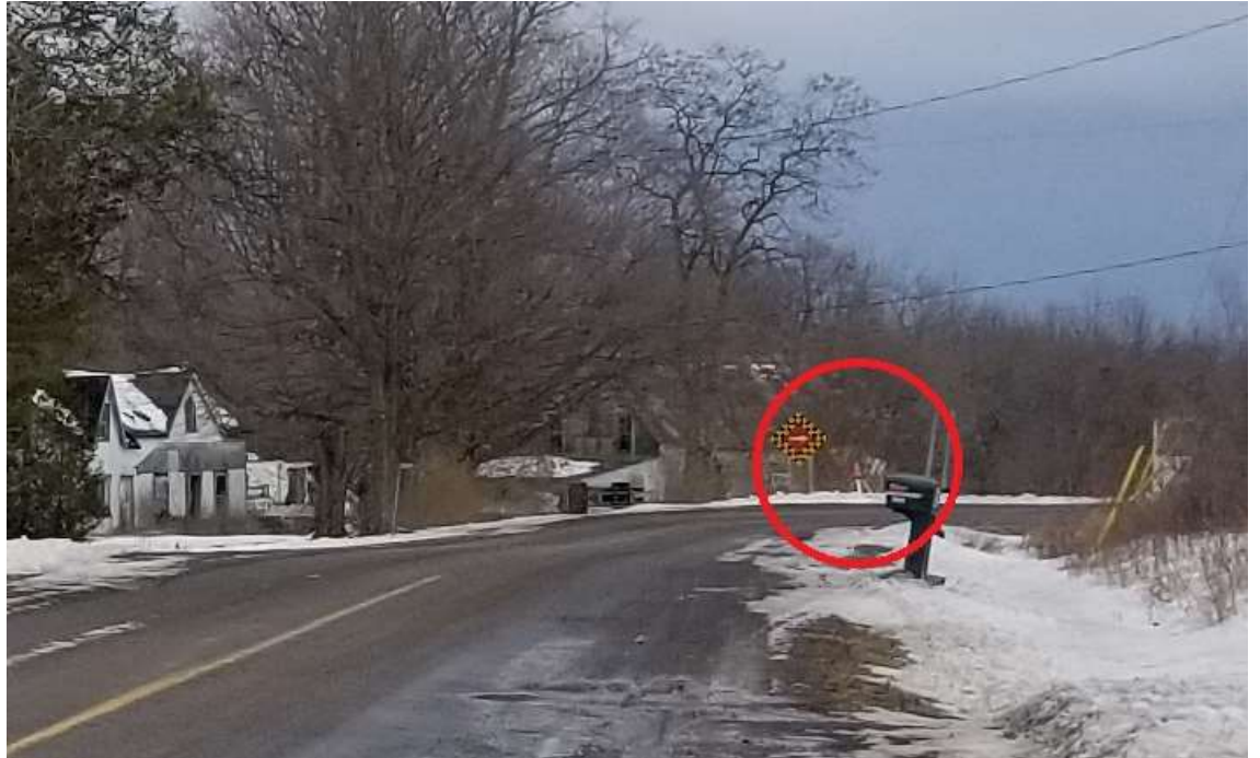
Looking eastbound toward access location A1 from 170m away
