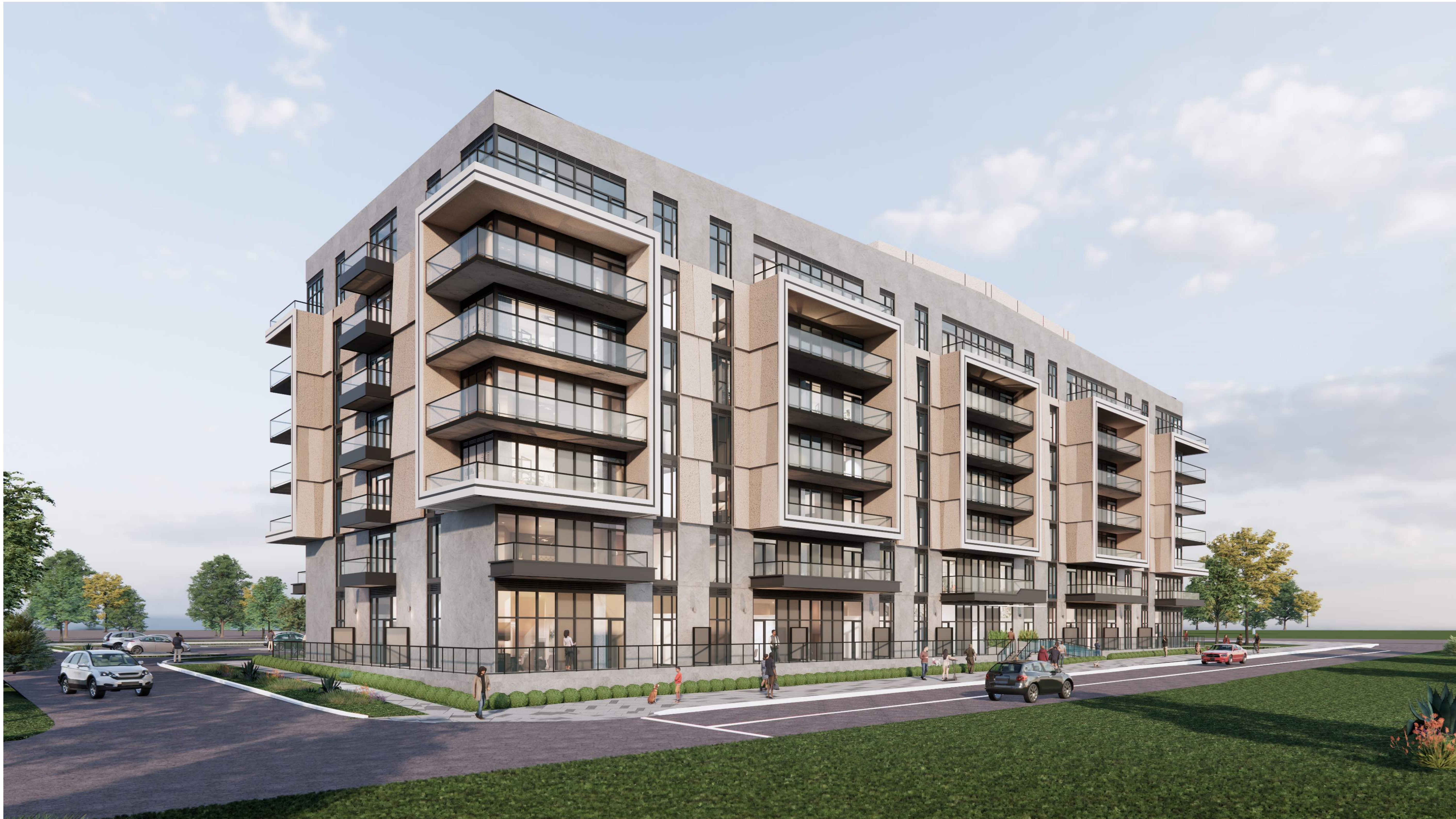
VIEW FROM CHURCH STREET LOOKING SOUTHWEST
