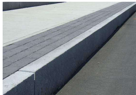
Splash pad adjacent sidewalk
