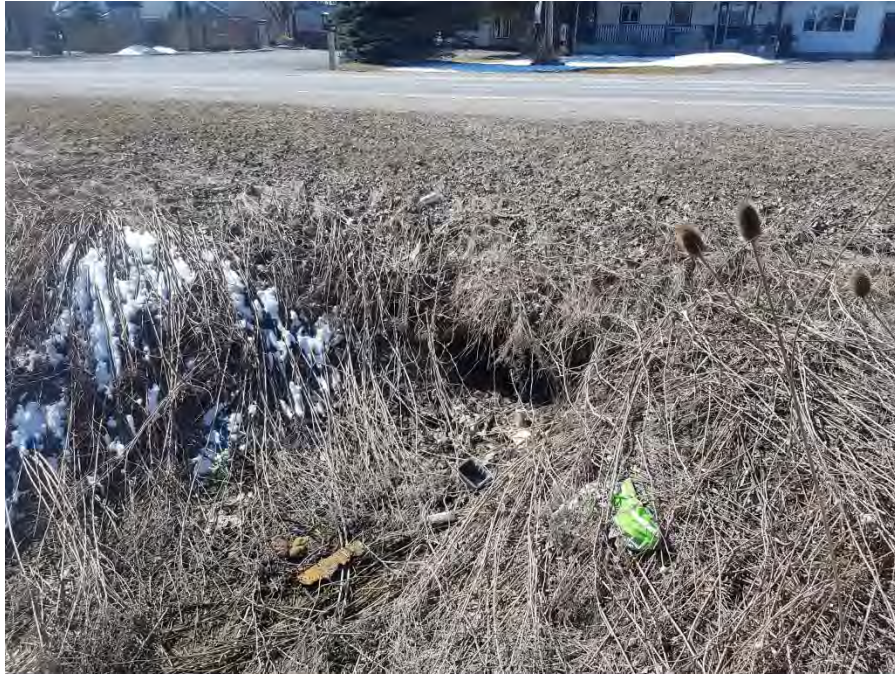
Photo 5 Culvert draining onto west side of Site
