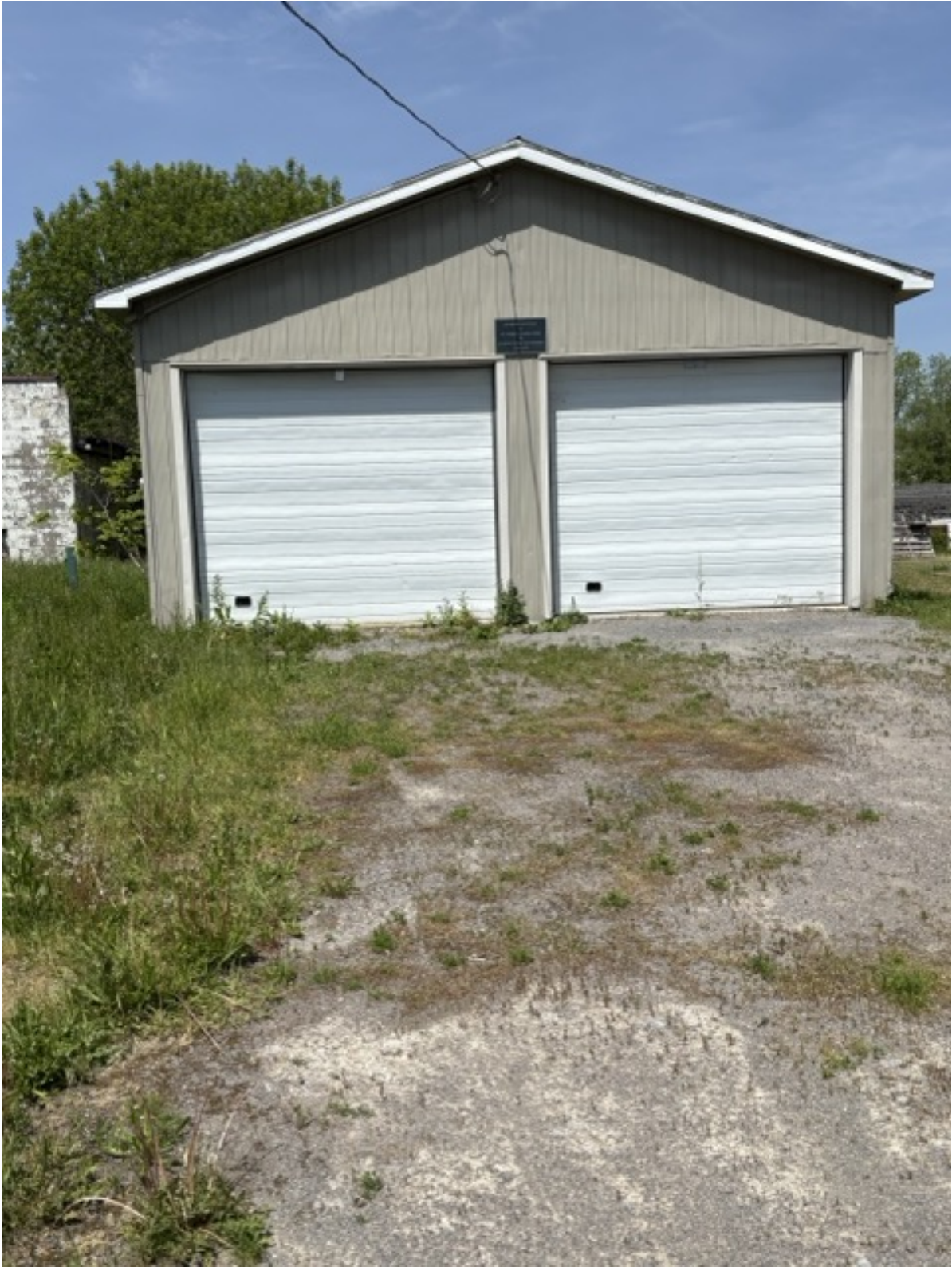
Photo taken from Consecon Street - Front of Building
