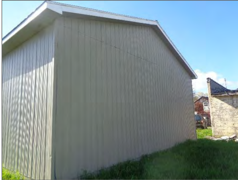
Photo 3 – West elevation of the Site Building, looking southeast.
