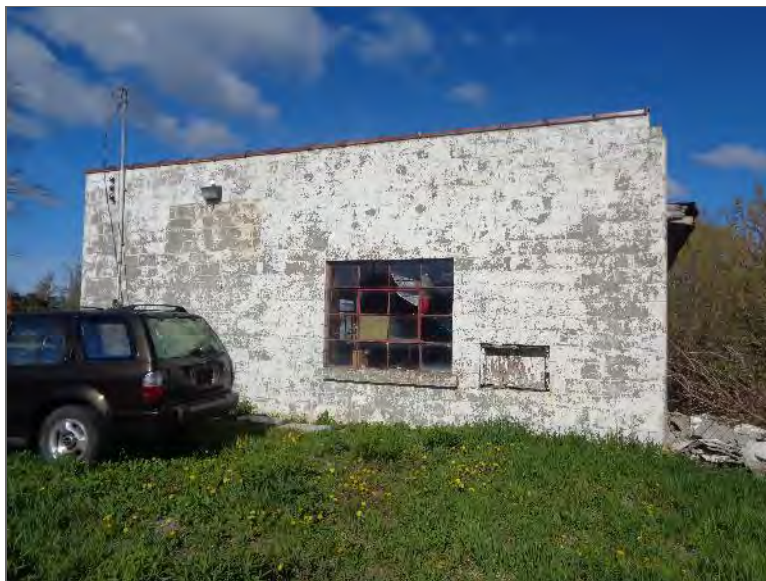
Photo 6 – South adjacent property (former automotive repair facility).
