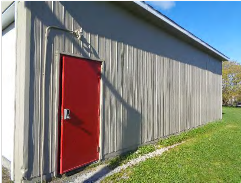
Photo 1 – North elevation of the Site Building, looking southwest.
