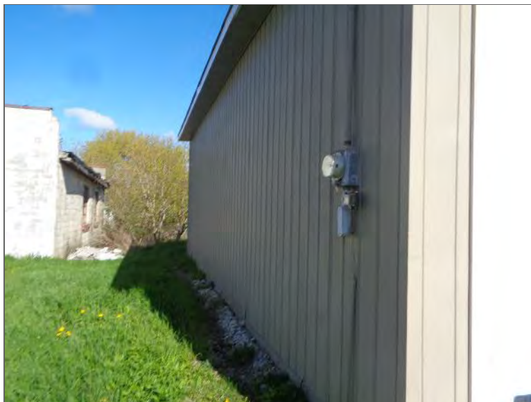
Photo 2 – South elevation of the Site Building, looking west.
