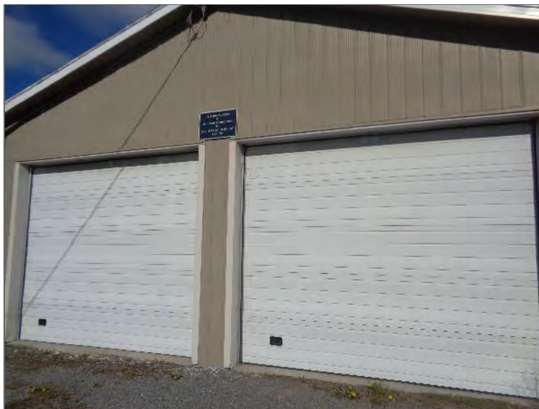
Photo 4 – East elevation of the Site Building, looking southwest.
