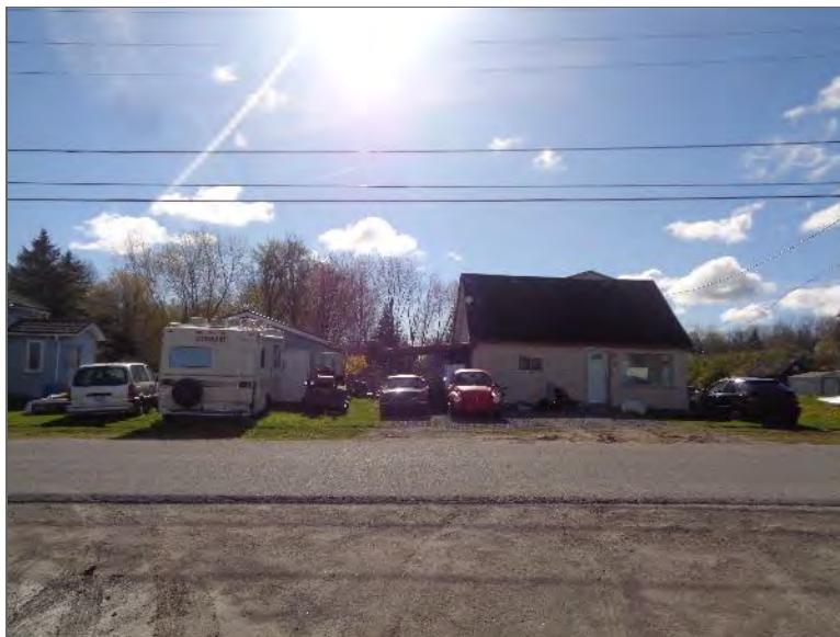
Photo 8 – East surrounding properties.
