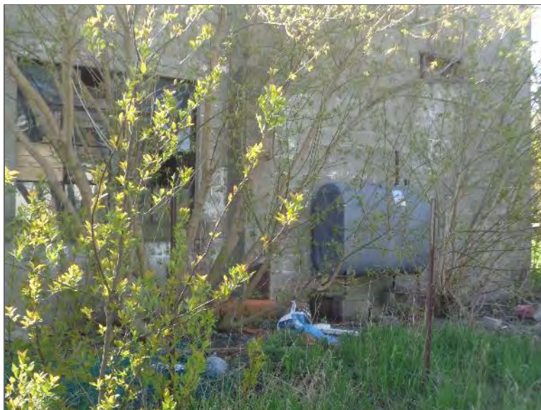
Photo 10 – South adjacent heating oil AST.
