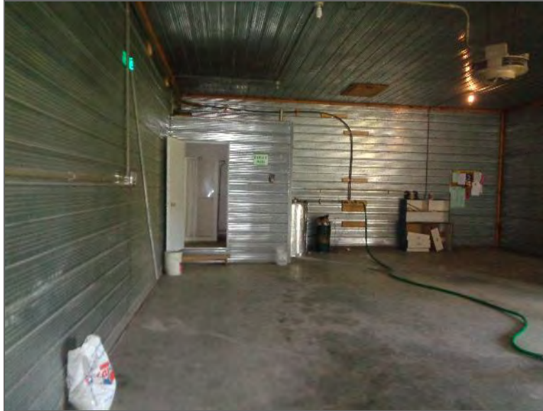
Photo 5 – Interior of Site Building.
