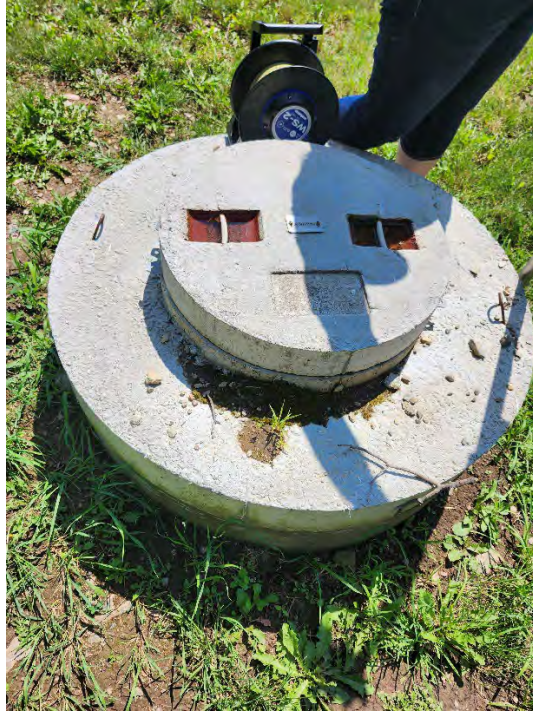
Photo 3: Monitored well A307989 on the retained lands that services a residential dwelling
