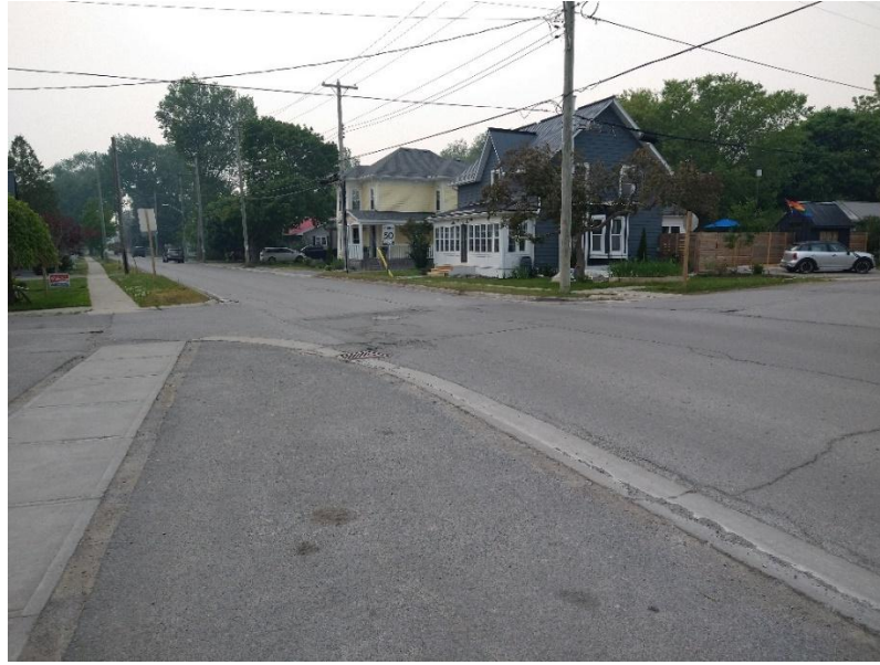
Figure 6-21: Main St at Consecon St Looking West
