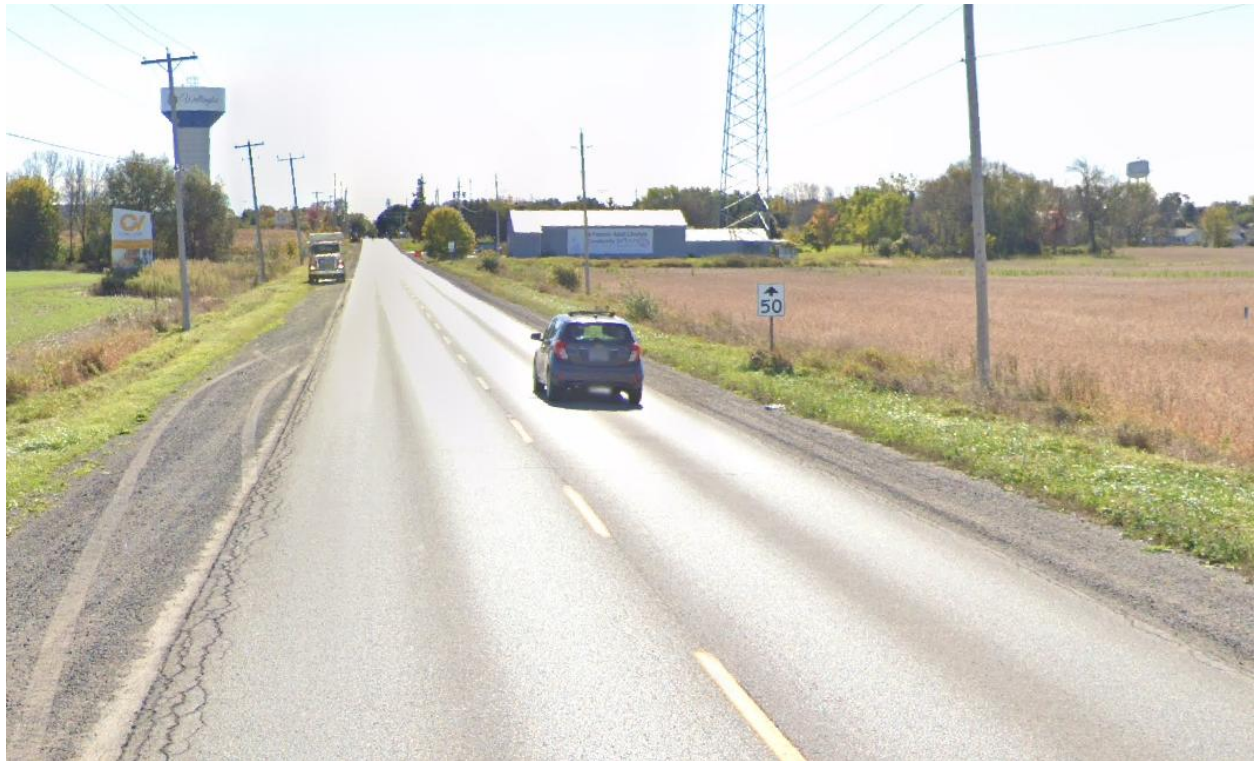
Figure 6-27: Belleville at Location of Turner St, Facing South (Google, Maxar Tech 2023)
