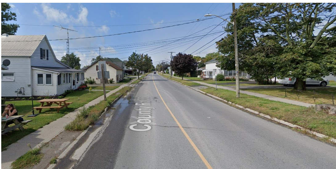
Figure 3-6: Wellington Main Street, Widened Westbound Lane (CR33) (Google, Maxar Tech 2021)
