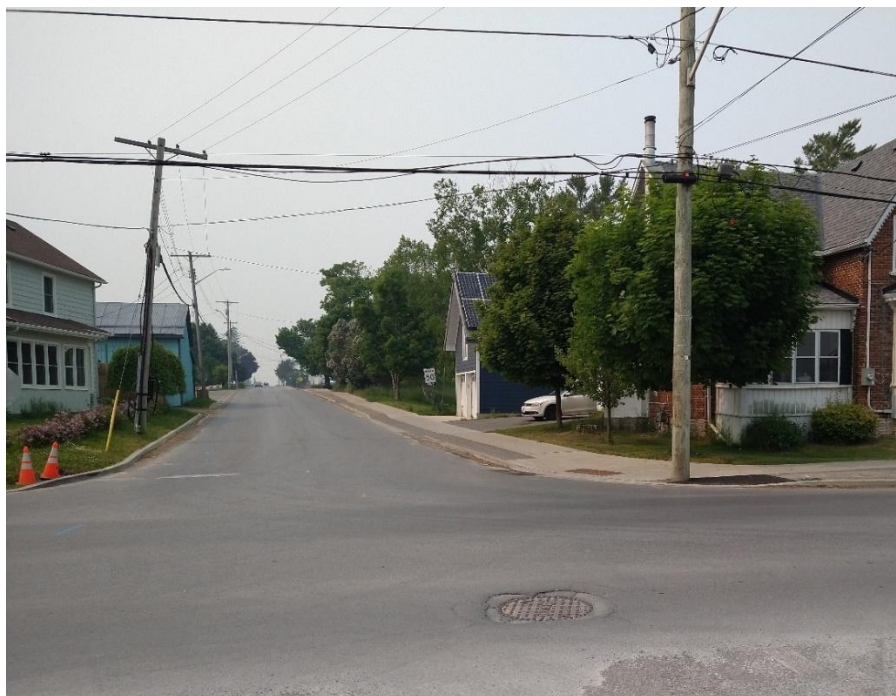
Figure 6-16: Belleville St Looking North (2023)
