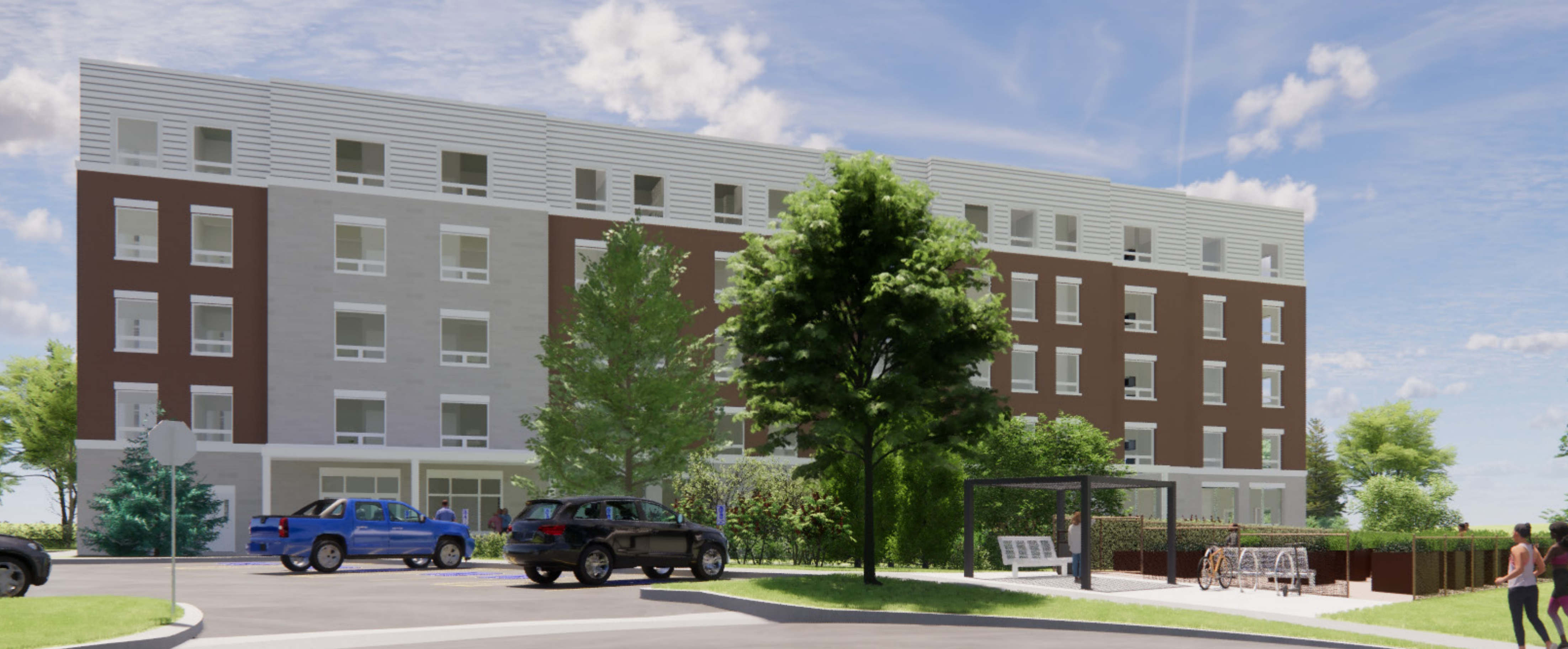
VIEW OF BUILDING D, INTERNAL TO SITE, LOOKING WEST
