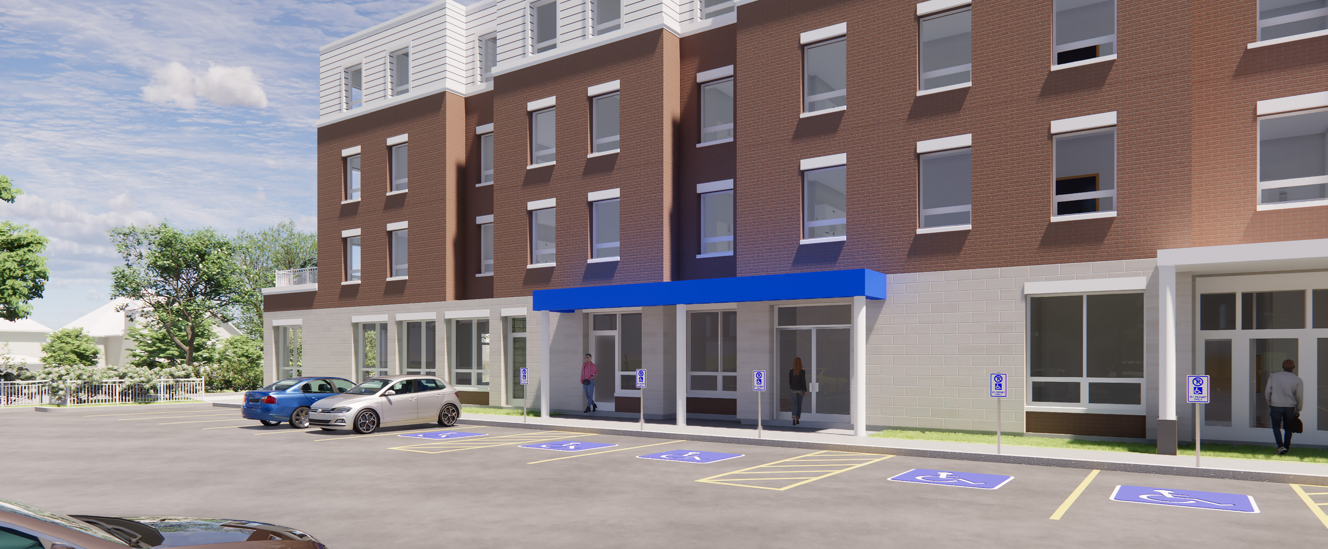
VIEW OF BUILDING A INTERNAL TO SITE, LOOKING EAST TOWARDS CENTRE STREET
