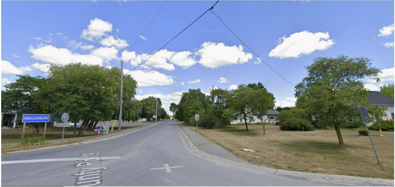
Intersection of Whitney Road and County Road 19 (pre-construction)
