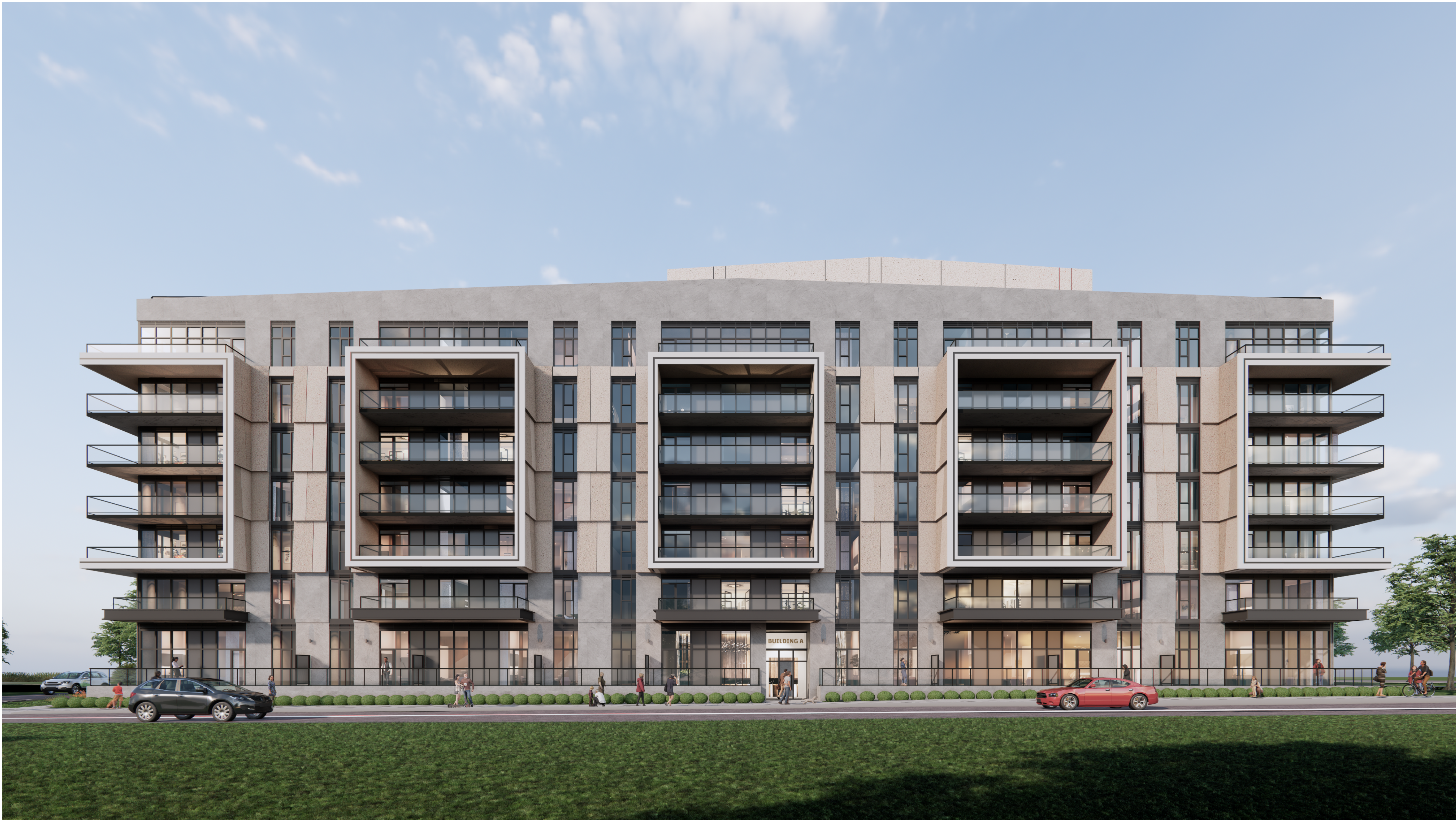
VIEW FROM CHURCH STREET LOOKING SOUTH
