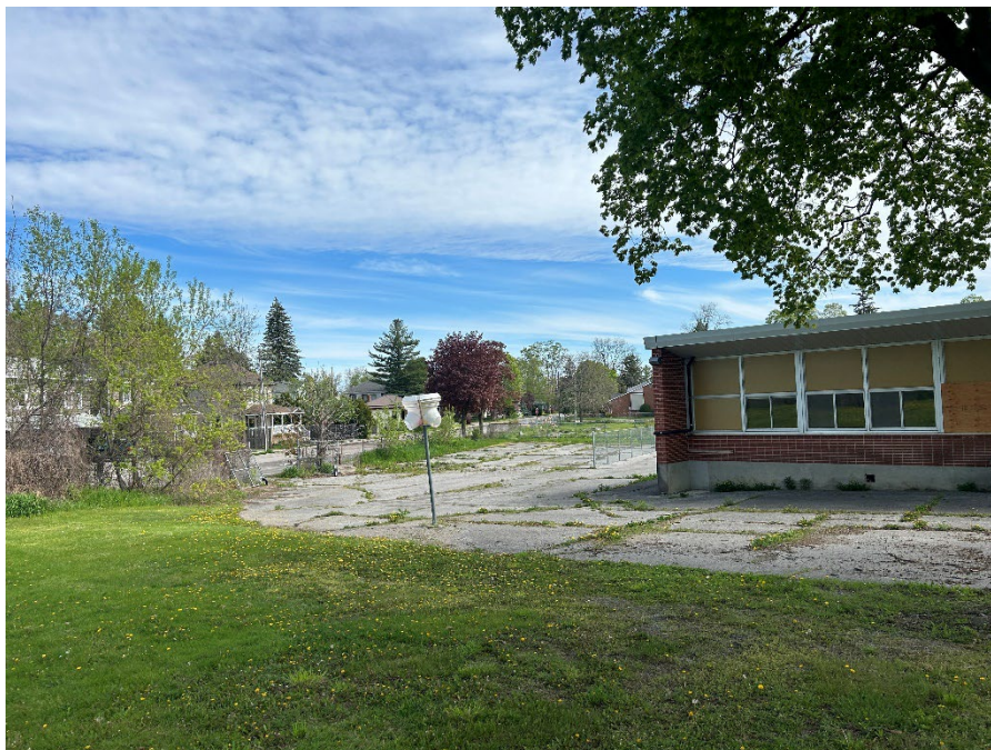
Photo 7 Northwest side of the Site, May 10, 2024.
