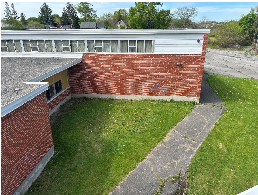
Photo 5 Northeast side of the Site Building, May 10, 2024.
