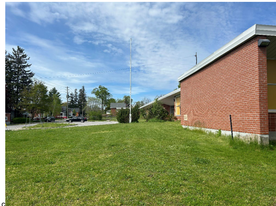
Photo 1 Southwest side of the Site Building, May 10, 2024.
