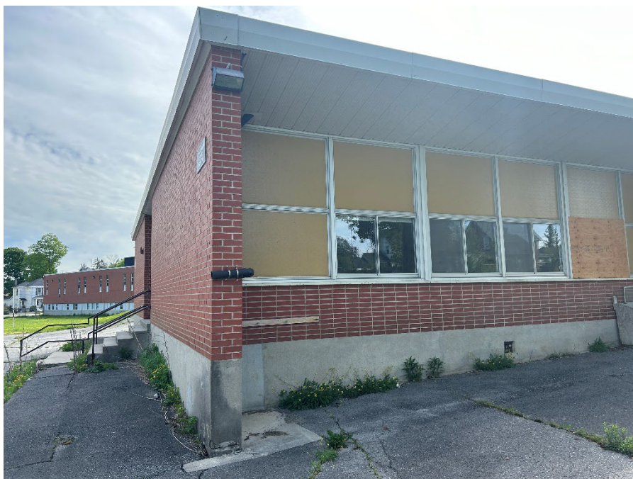
Photo 2 Northwest side of the Site Building, May 10, 2024.
