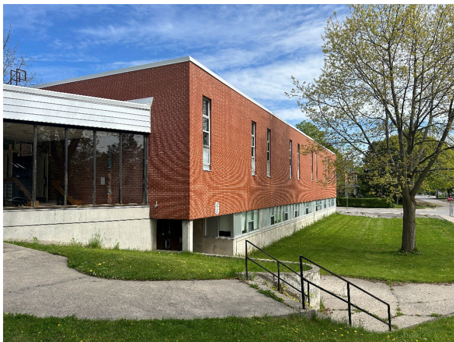
Photo 4 Southeast side of the Site Building, May 10, 2024.
