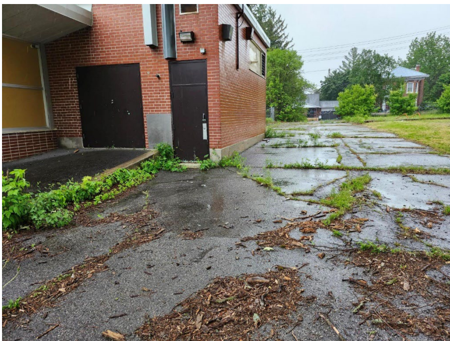
Photo 8 Location of former UST, southwest portion of the Site Building, May 27, 2024.
