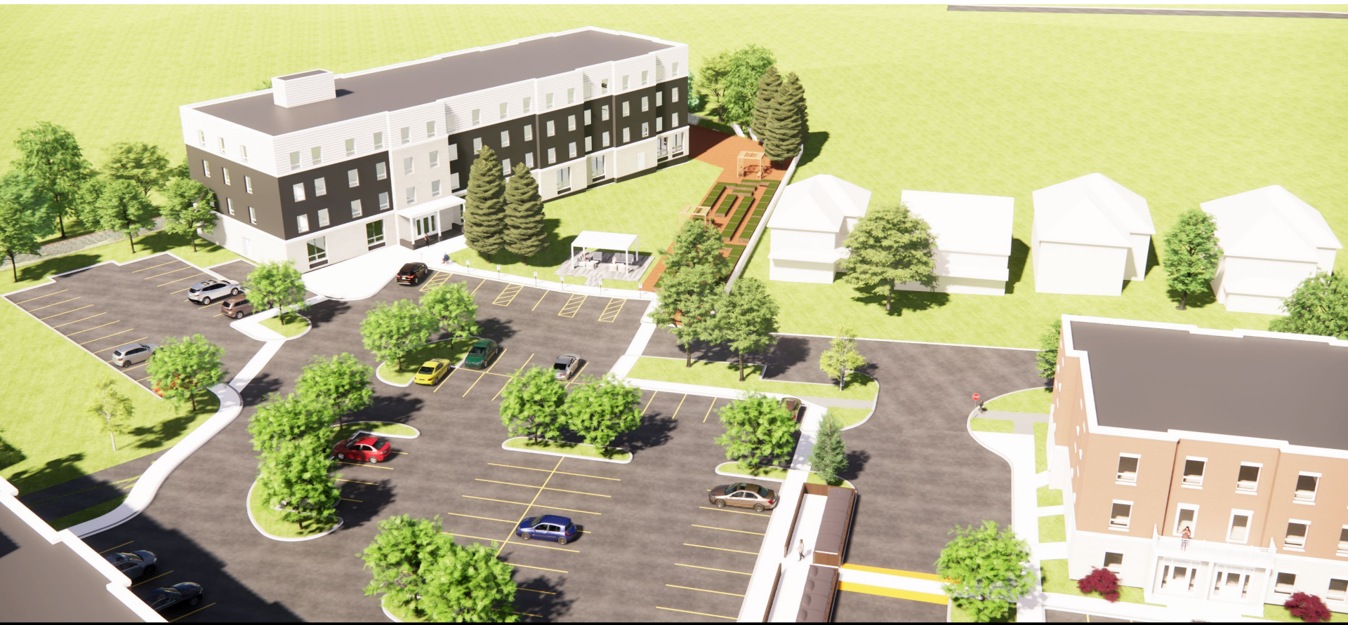
VIEW INTERNAL TO SITE OF BUILDING D, COMMUNITY GARDEN, AND BUILDING B
